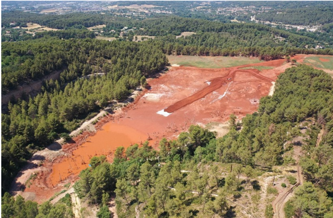
Figure 5. Overall view of pond 7 at the start of the works.
