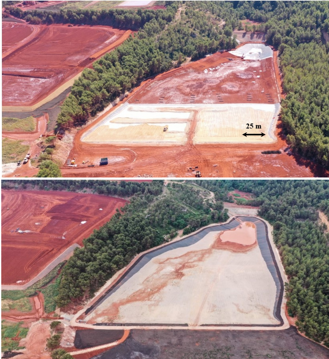
Figure 7. Overview of the rainwater collection pond sealing project.
