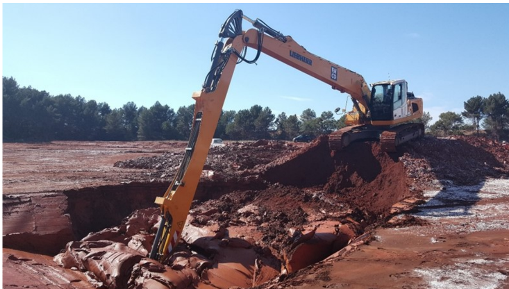
Figure 4. Digging test with a long reach excavator.
